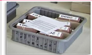
A tile tub with tiles sorted and ready for placement
