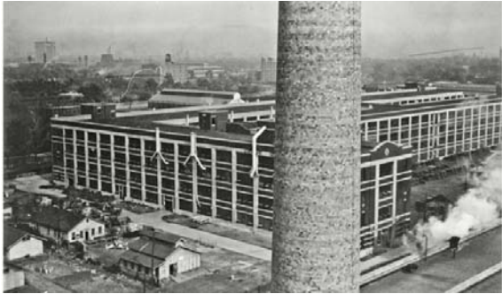
Clark Street Plant
